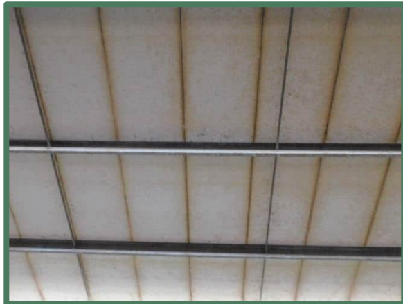
Dak van sandwichpanelen
